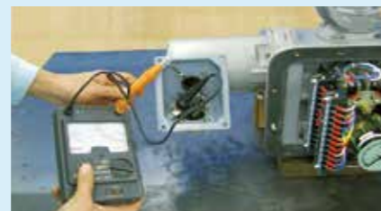
Electrical insulation measurement
